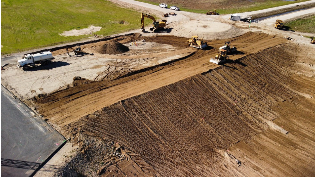
Figure 2 – GSE Construction’s subcontractor Damar Construction performing rough grading for Iron and Manganese Treatment Plant project site
