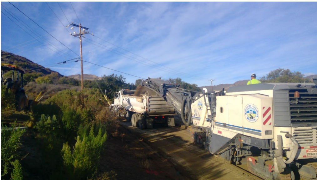
Figure 1 – Removal of the existing road base material at Lake Piru Water Treatment Plant
