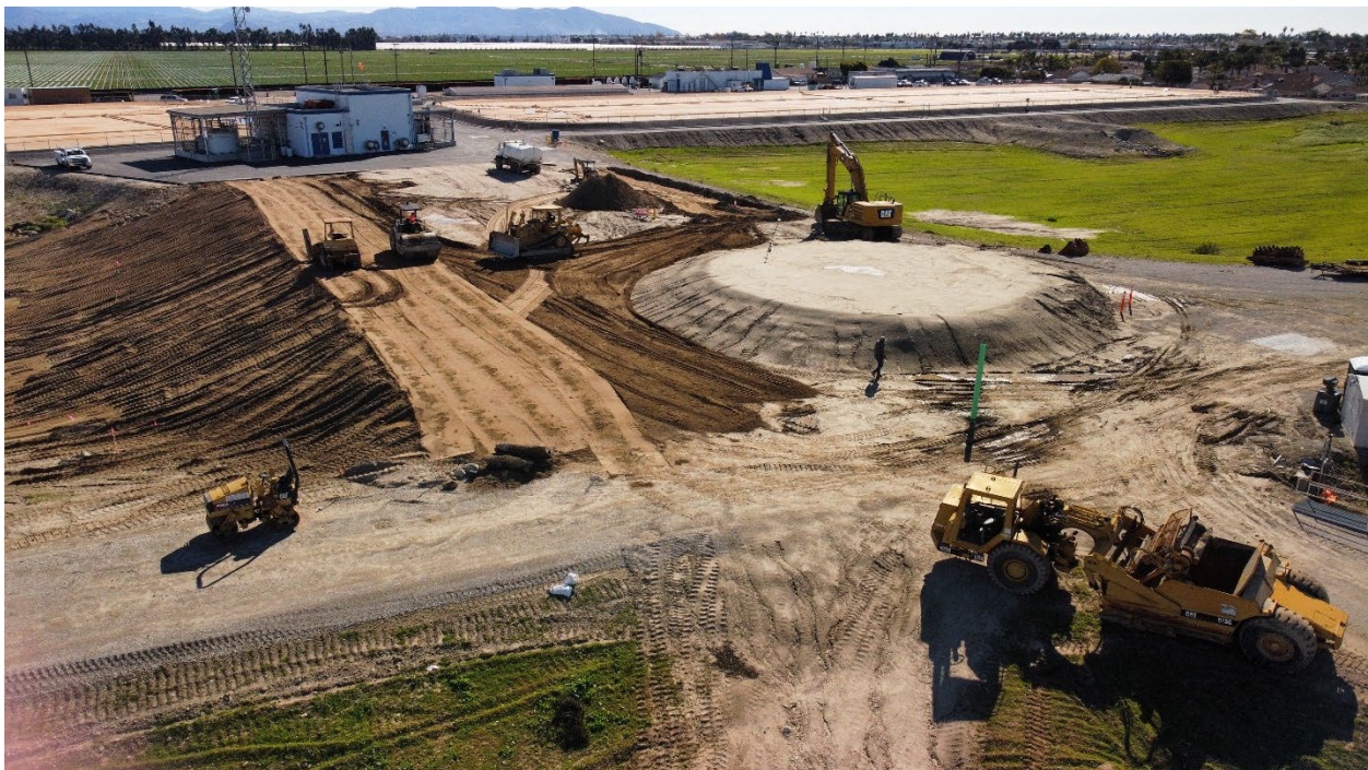
Figure 3 – GSE Construction’s subcontractor Damar Construction building up washwater recovery tank pad for Iron and Manganese Treatment Project
