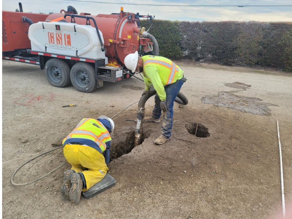
Figure 4 – GSE Construction crew performing vacuum potholing of utility crossing with proposed sewer line and back wash supply pipeline
