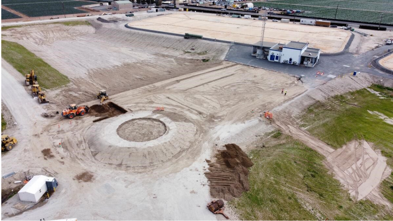
Figure 1 - Rough Grading in Pond 8 complete. Excavation for installation of Filter Drain Pump Station underway (photo taken Jan 13, 2022)
