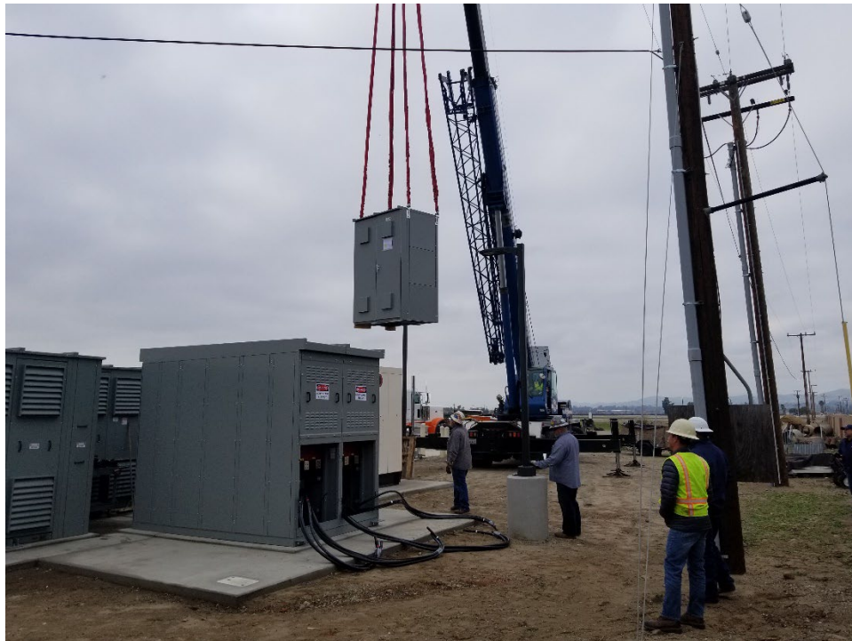
Figure 4 - OH System Backup Generator Project - Installation of Medium Voltage Switches (photo taken Jan 19, 2022)
