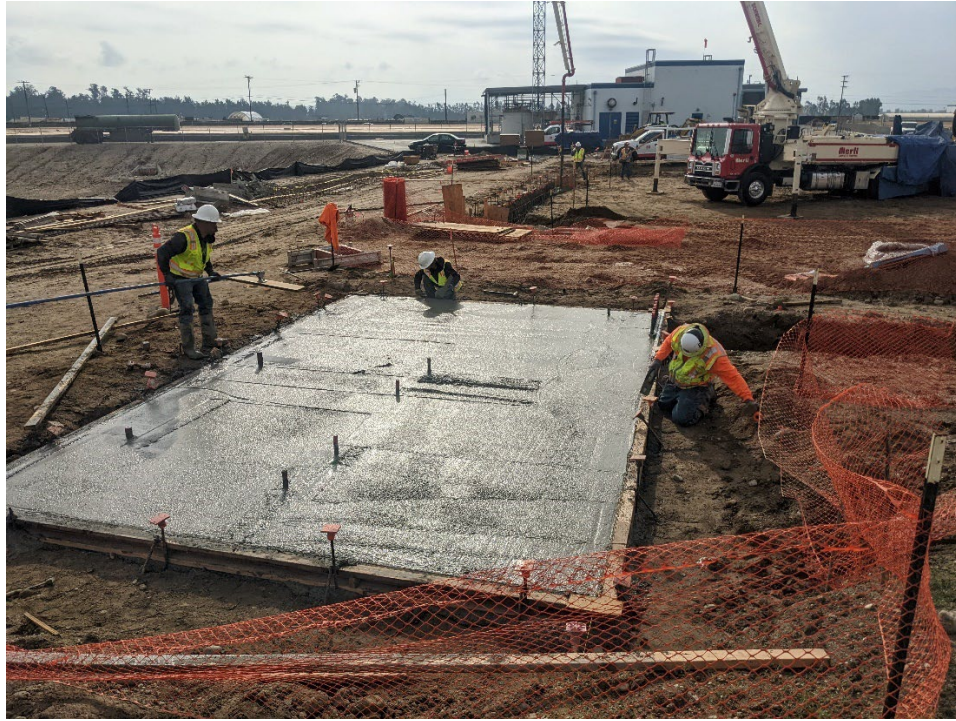
Figure 3 – Washwater Return Pump Station Concrete Placement on March 31
