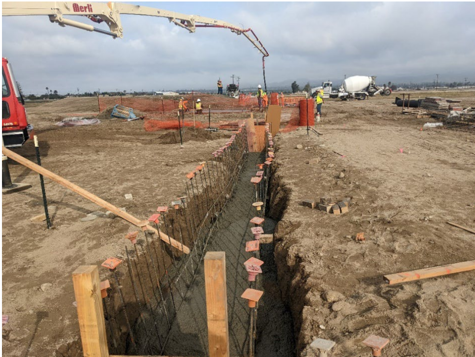
Figure 4 – Surface Wash Water (SWW)/Filter to Drain (FTD) Concrete Encasement Placement on March 31
