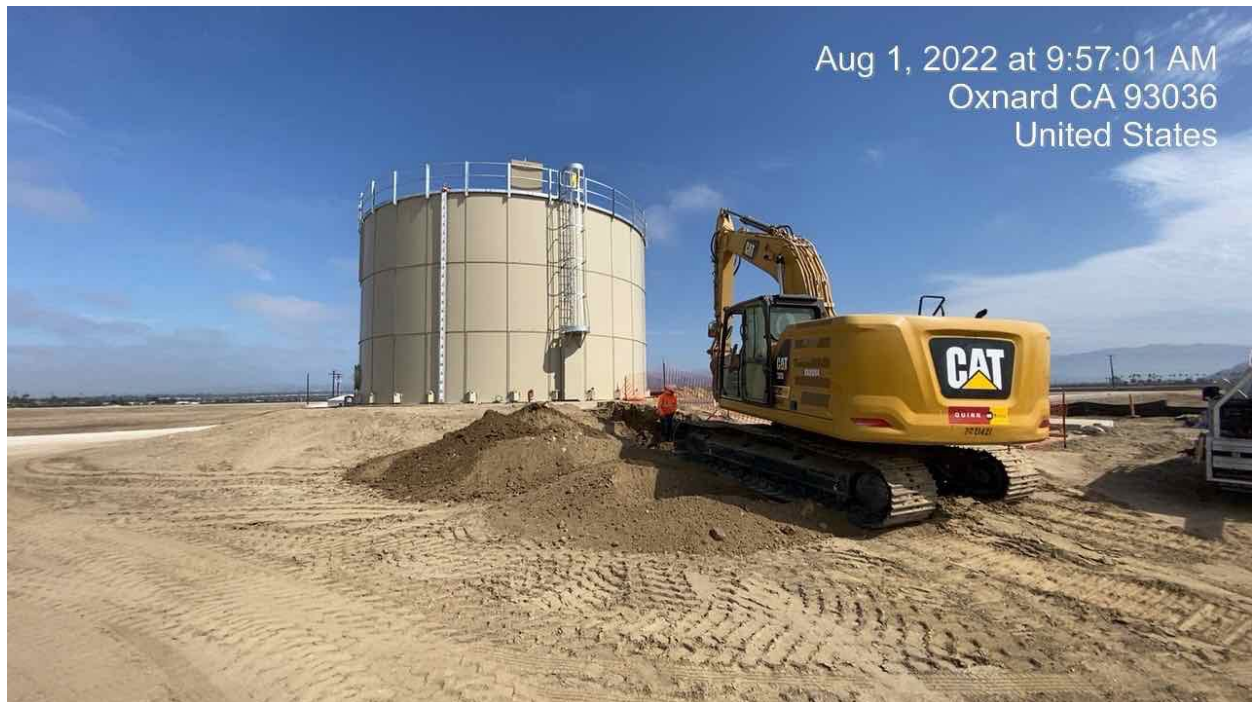
Figure 1 – Washwater Recovery Tank at the new Iron and Manganese Treatment Plant
