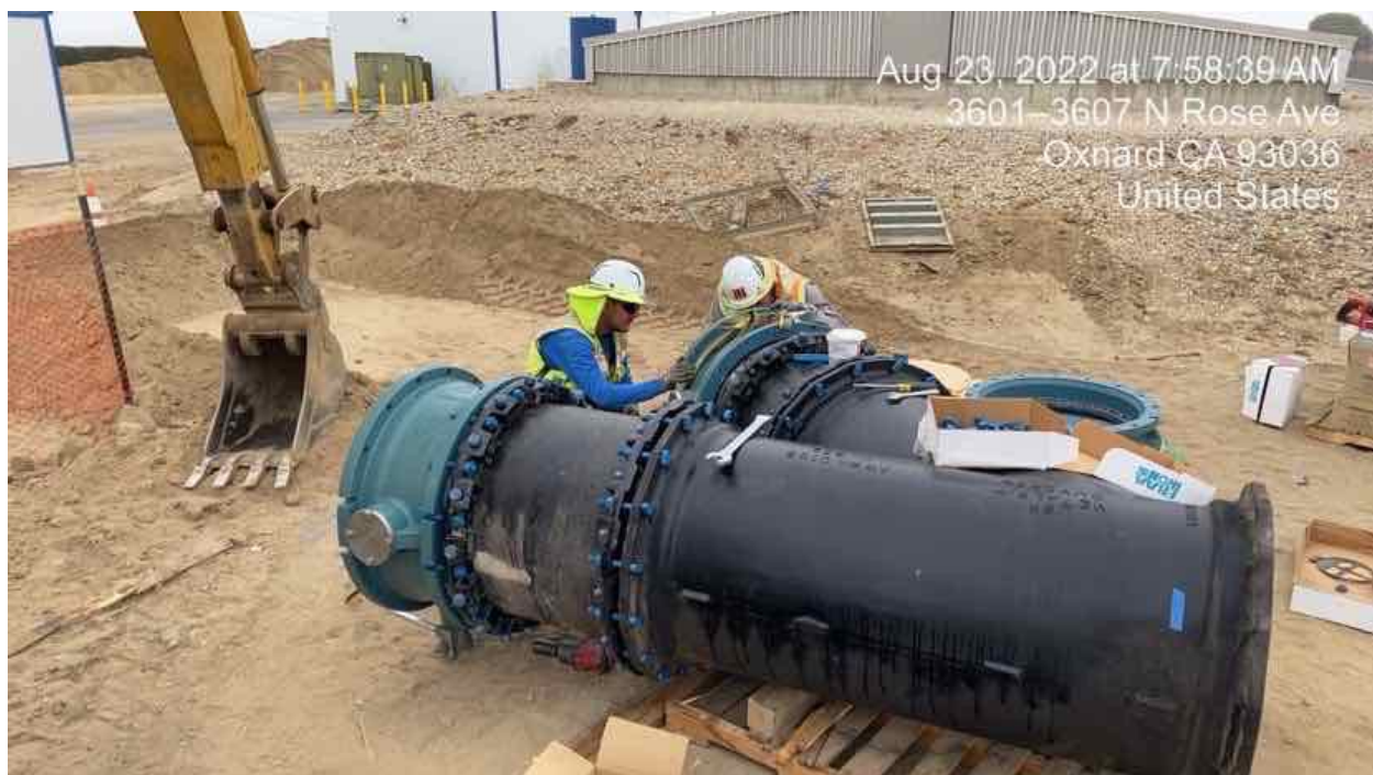
Figure 4 – GSE Construction staff assembling 24” raw water pipeline manifold valves that will supply water from El Rio Well Nos. 12, 13 and 14 to the new Iron and Manganese Treatment Plant
