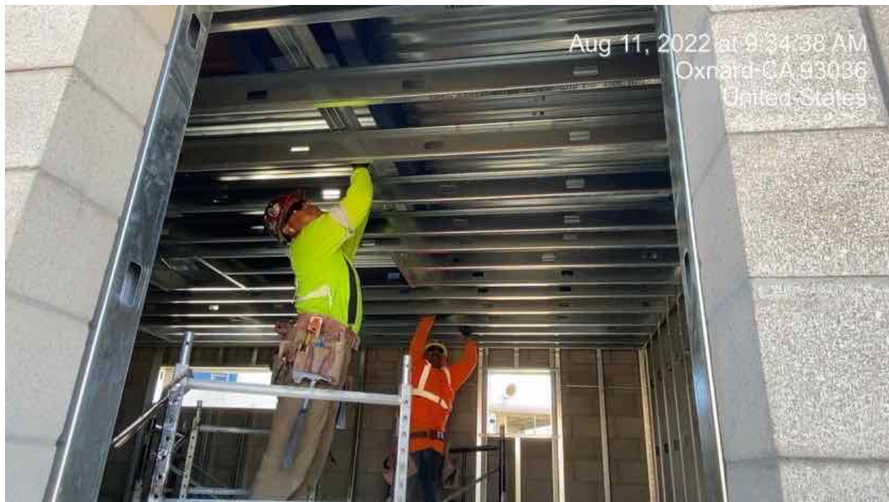
Figure 3 – GSE Construction’s subcontractor Tarlton and Son’s installing internal framing inside the laboratory room at the Iron and Manganese Treatment Plant.
