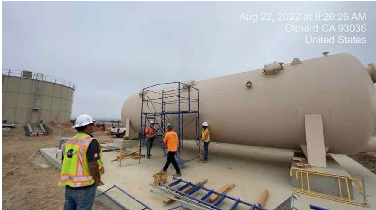
Figure 2 – GSE Construction prepare scaffolding for access into Filter Vessel #1.
