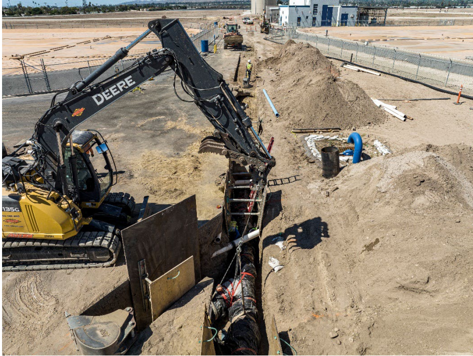
Figure 2 – RAW pipeline under construction as part of the Iron and Manganese Treatment Project (connects the new treatment plant to Well Nos. 12, 13 and 14)
