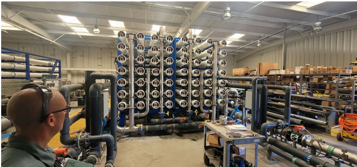
Figure 5 – Tour with Navy staff of the PHWA BWRDF. Two treatment skids shown including Nanofiltration (left) and Reverse Osmosis (right).
