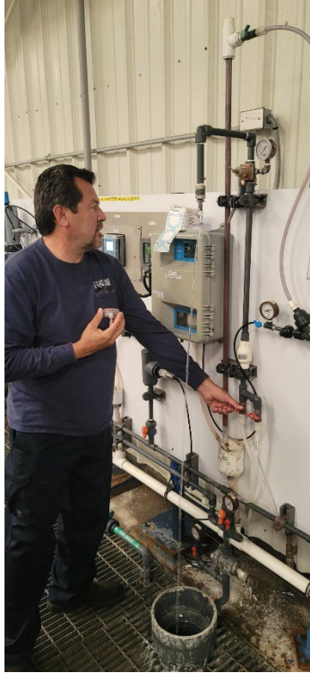
Figure 6 – Theo Provencio (Lead Operator) demonstrates Silt Density Index (SDI) sampling during a tour of the PHWA BWRDF.
