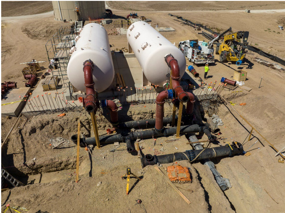
Figure 3 – Filter face piping under construction as part of the Iron and Manganese Treatment Project
