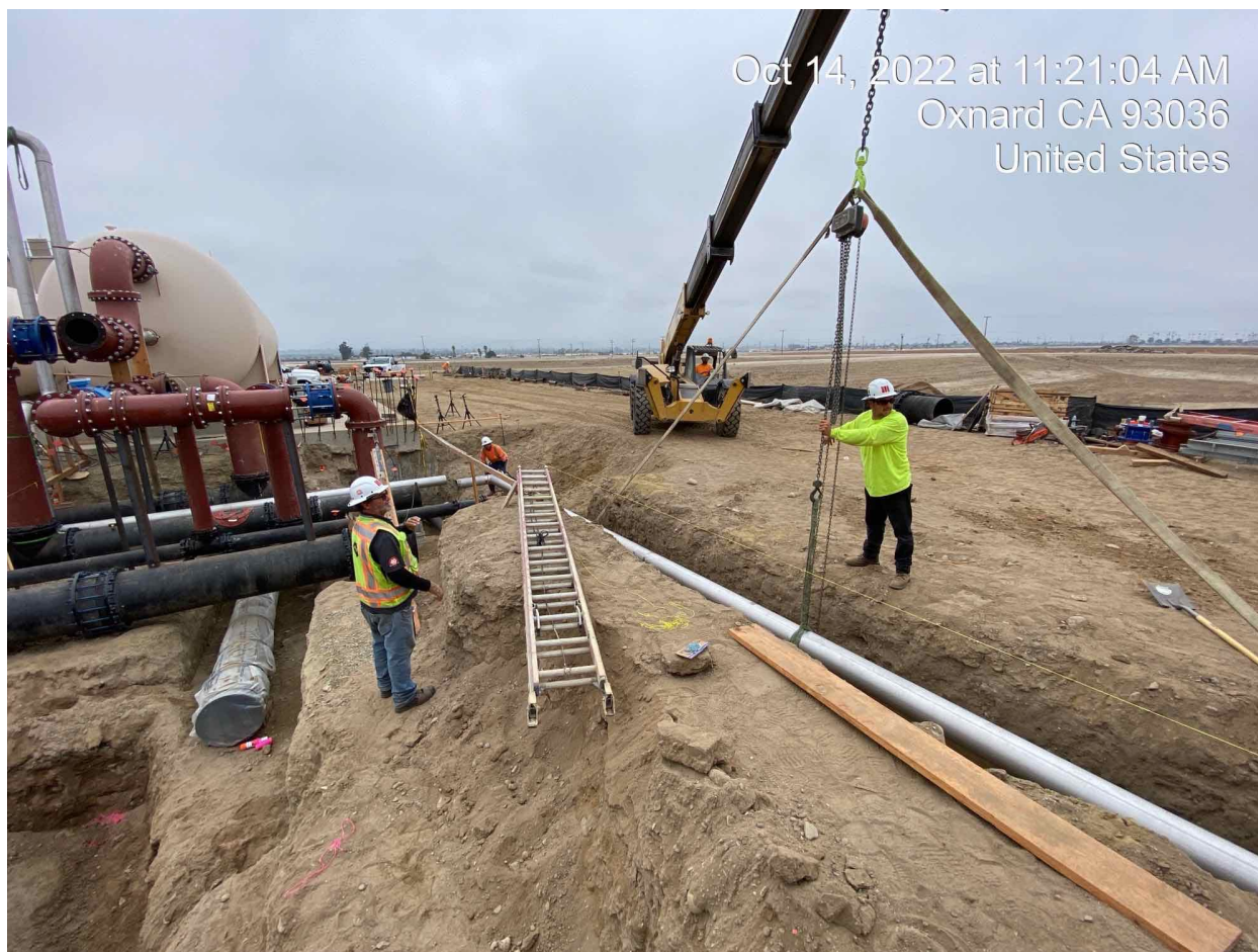
Figure 1 - 8" Welded Stainless Steel Air Supply Pipeline Installation
