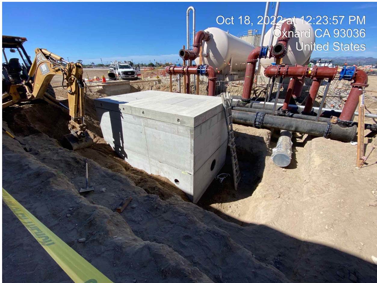
Figure 3 - New Backwash Supply Vault and Filter Face Piping
