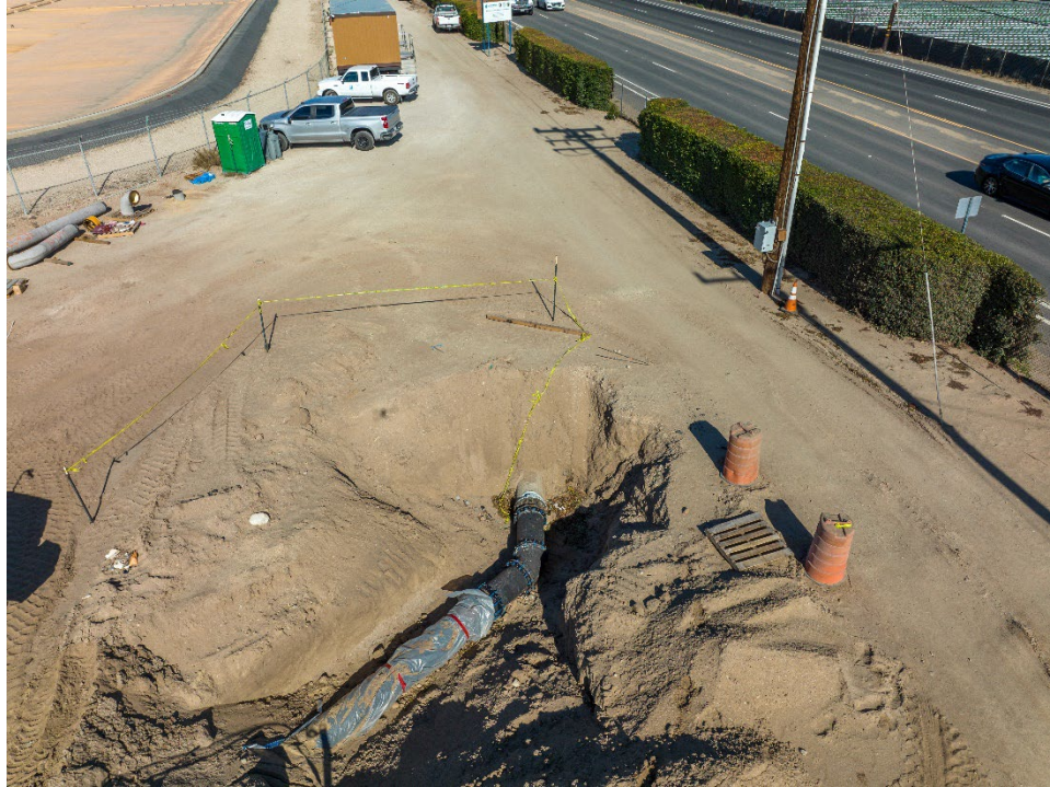
Figure 7 – RAW Pipeline Tie-In to Well 12 and 13 Manifold
