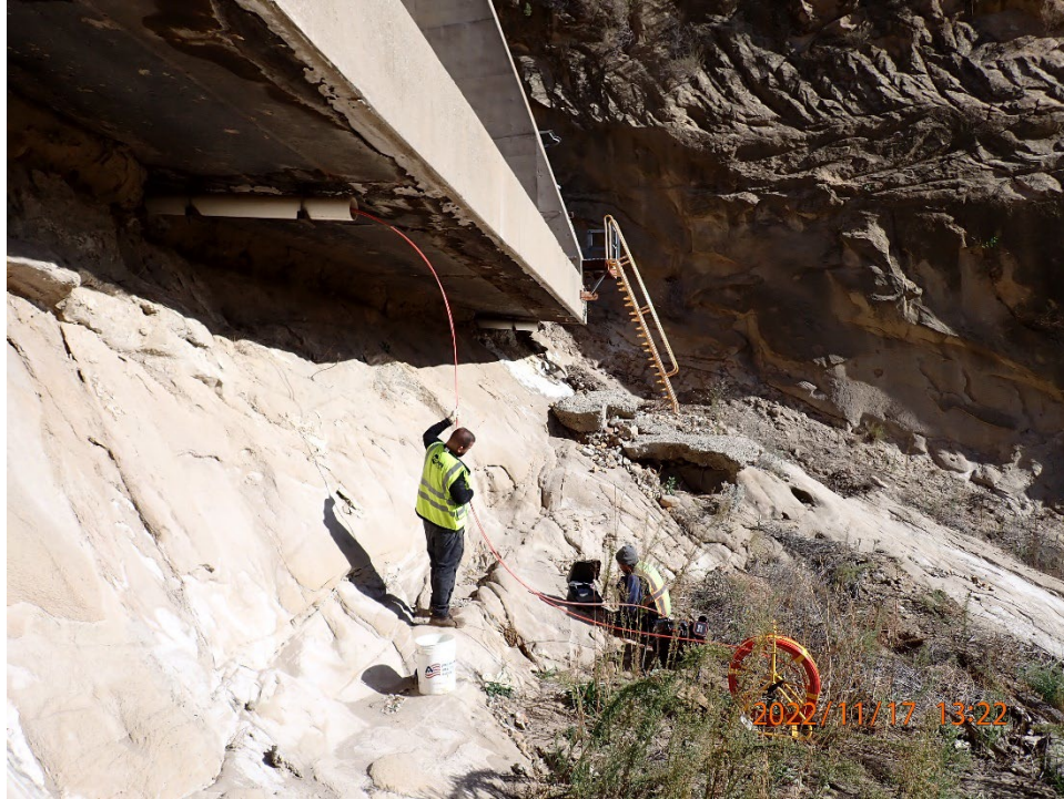
Figure 3 – Santa Felicia Dam Spillway Underdrain Inspection
