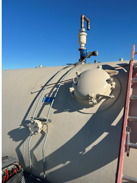
Figure 3 – Installation of 3” Electrically Actuated Valves on Filter Vessel Vents
