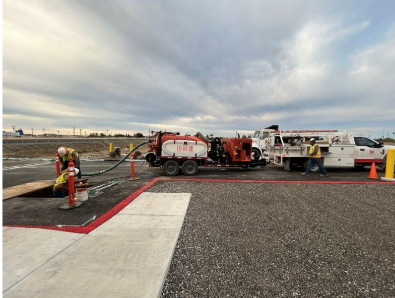
Figure 5 – GSE Construction Vacuum Excavating at Buried 24” Butterfly Valve
