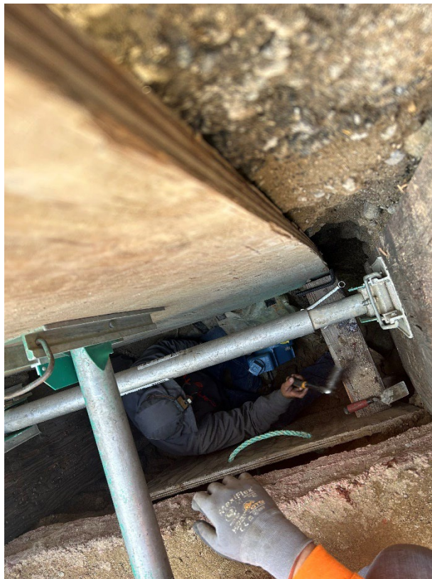
Figure 6 – GSE Construction Replacing Gearbox at Buried 24” Butterfly Valve
