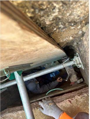
Figure 6 – GSE Construction Replacing Gearbox at Buried 24" Butterfly Valve
