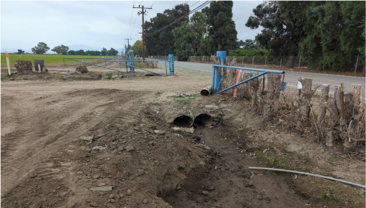
Photograph 17. View of culverts associated with Ditch 2 in the western portion of the Study Area (Aspect: southeast; September 13, 2023).
