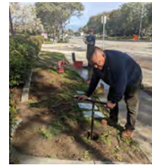
Fire Sprinkler Inspection on February 16
