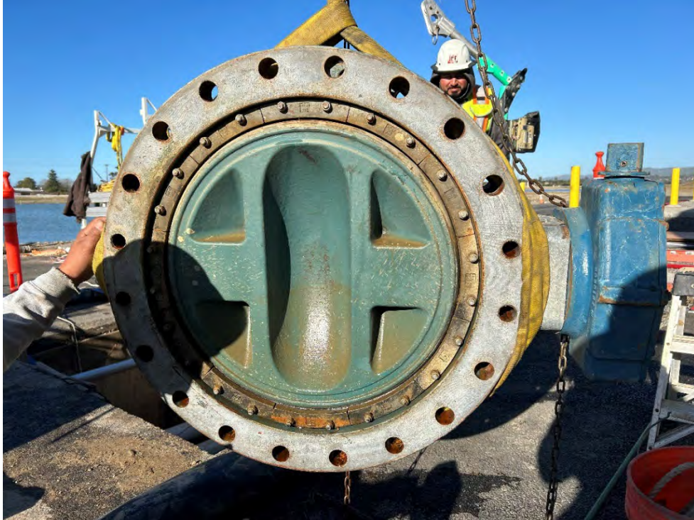
Figure 1 – 24” FW Butterfly Valve Removal at Fe/Mn Plant
