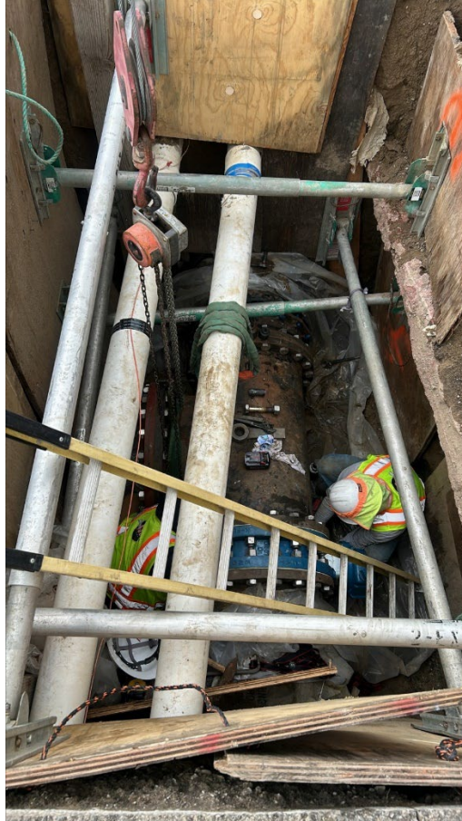
Figure 1 – Installation of Refurbished 24” FW Valve.
