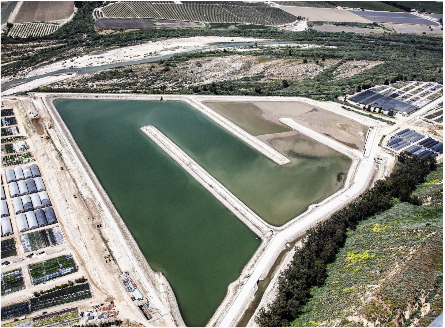
One of United's recharge basins.
