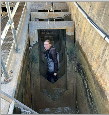
Freeman Fish Ladder Operations
