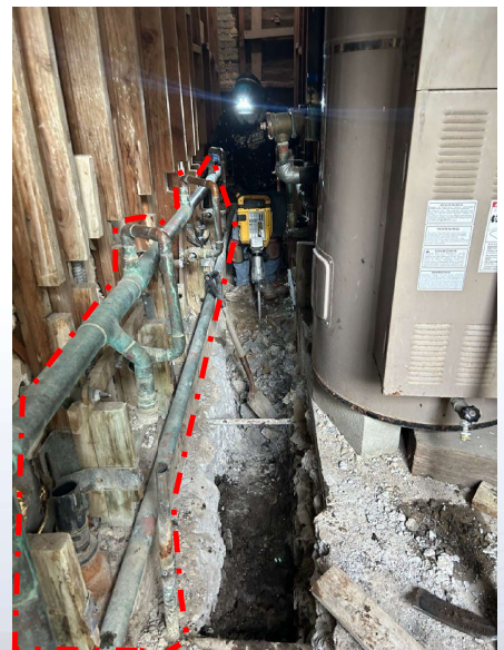
Waterline relocation Additional concrete demolition
