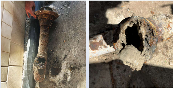
Condition of floor drains
