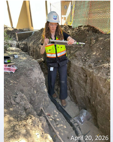
Checking sewer slope before inspection and testing
