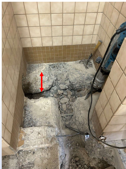
Additional concrete demolition
