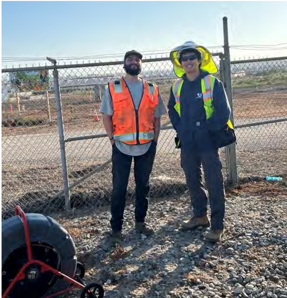
Figure 1: September 3 - Associate Engineer Matt Wong attending the Well 14 discharge head and pipeline camera inspections by GPRS
